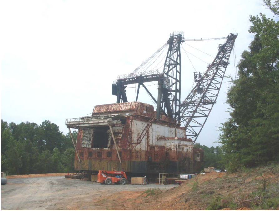
Figure 5. Current Location of Dragline in Section 4.
