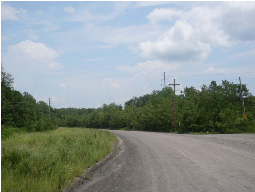
Figure 12. Access Road in Section 28 Leading to Quarry.
