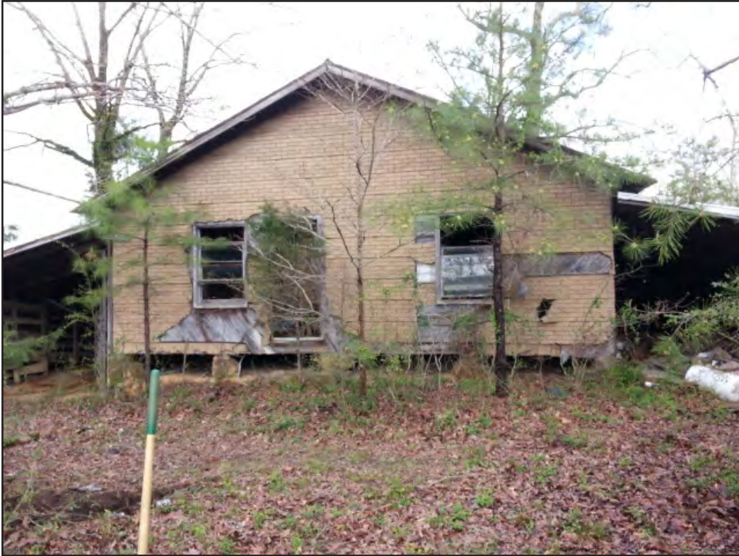
Figure 6. View of Structure 1 (Burton House), looking north.
