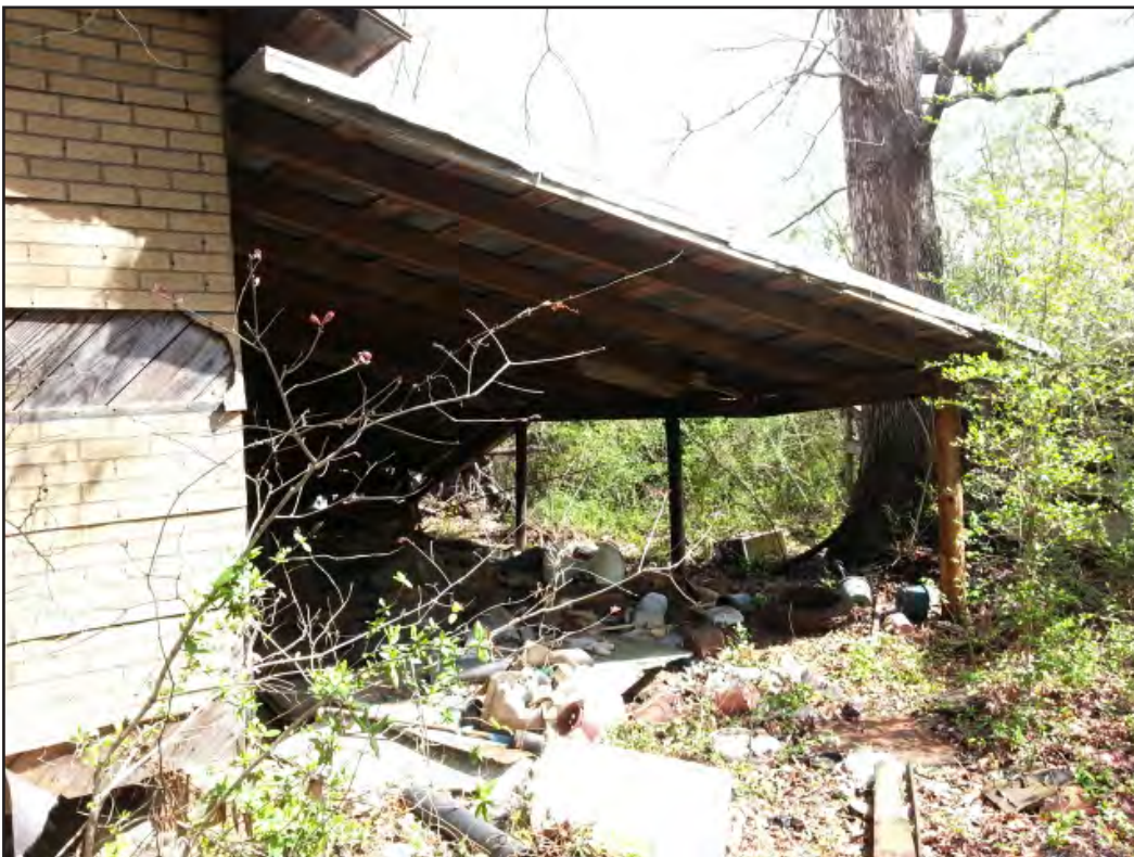
Figure 7. View of Structure 1 (Burton House) garage, looking northeast.
