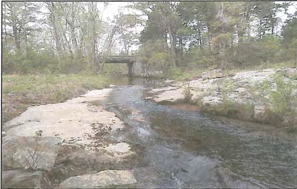
CRANE CENTRAL MINE SITE, 04 19 2016: Long Creek a short distance north of proposed site, view upstream of creek flow under County Road #14, sandstone bedrock creek bed. GPS N 34 50.577. W 085 43.008.
