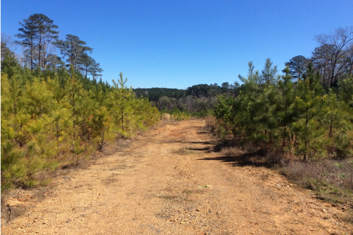
Figure 34. View to East of Dragline Route.
